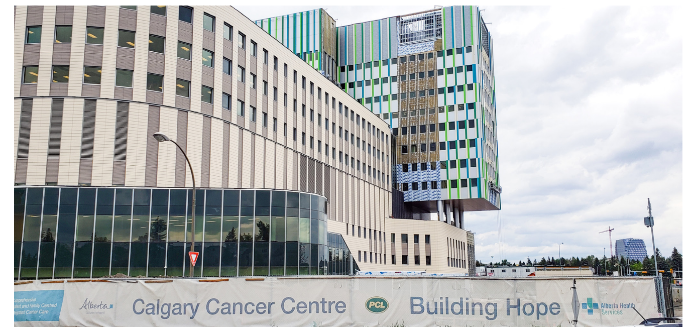
Image 5: Calgary Cancer Centre under construction, June 2021
